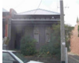
Carlton North Fenwick Street 166
