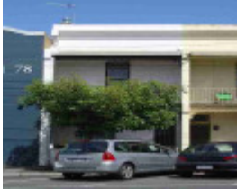
richmond docker street richmond docker street 74
