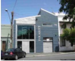
richmond docker street richmond docker street 78
