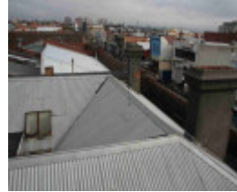
Collingwood Johnston Street 31-33 rear.JPG
