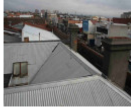
Collingwood Johnston Street 31-33 rear.JPG
