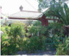
carlton north amess street carlton north amess street 201
