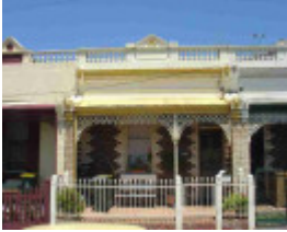
carlton north davis street carlton north davis street 41
