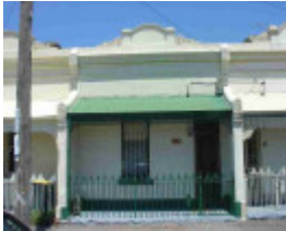
carlton north davis street carlton north davis street 47
