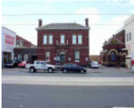
Richmond Police Station
