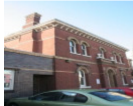
Richmond Police Station
