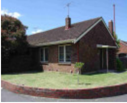
burnley bridge road burnley bridge road 634
