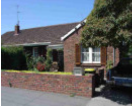
burnley bridge road burnley bridge road 638
