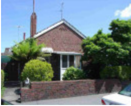
burnley bridge road burnley bridge road 640
