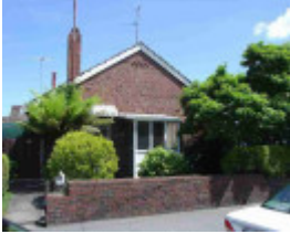
burnley bridge road burnley bridge road 640
