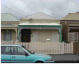
richmond cotter street richmond cotter street 37
