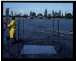
ALBERT PARK LAKE EXCAVATION
