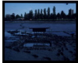
ALBERT PARK LAKE EXCAVATION
