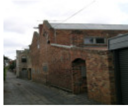
Store - Rear 141 Pigdon (west elevation).JPG
