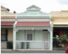
princes hill holtom street princes hill holtom street 87
