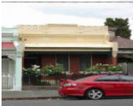
princes hill holtom street princes hill holtom street 89
