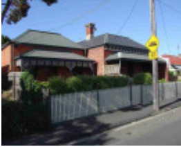
richmond lesney street richmond lesney street 34
