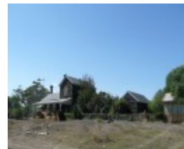
BANNOCKBURN RAILWAY STATION SOHE 2008
