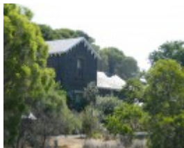
BANNOCKBURN RAILWAY STATION SOHE 2008
