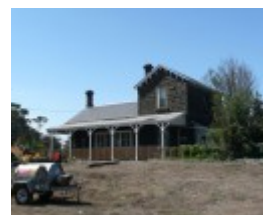
BANNOCKBURN RAILWAY STATION SOHE 2008
