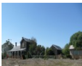
BANNOCKBURN RAILWAY STATION SOHE 2008
