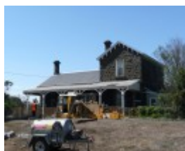
BANNOCKBURN RAILWAY STATION SOHE 2008
