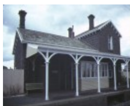
1 bannockburn railway station rear elevation aug1984
