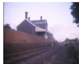
bannockburn railway station side view apr1995
