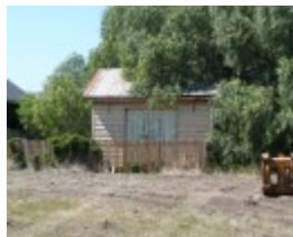
BANNOCKBURN RAILWAY STATION SOHE 2008
