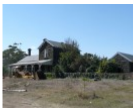
BANNOCKBURN RAILWAY STATION SOHE 2008
