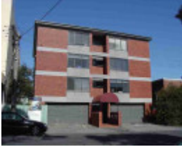
richmond lennox street richmond lennox street 263- 265 unit 1
