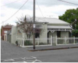
princes hill holtom street princes hill holtom street 101
