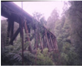
rail bridge noojee side elevation
