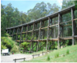
RAIL BRIDGE SOHE 2008
