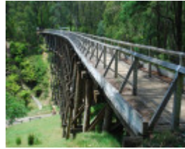
RAIL BRIDGE SOHE 2008
