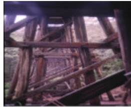
rail bridge noojee trestle view
