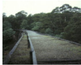
rail bridge noojee top view may1990
