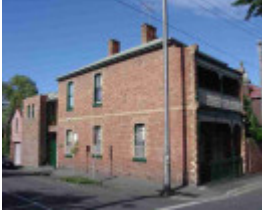
richmond lesney street richmond lesney street 24
