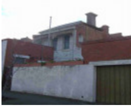
Carlton North Drummond Street 742 rear - facing Fenwick Street
