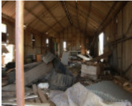
Clean-up re. asbestos 2012
