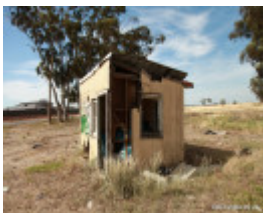
Clean-up re. asbestos 2012
