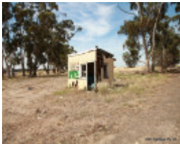
Clean-up re. asbestos 2012
