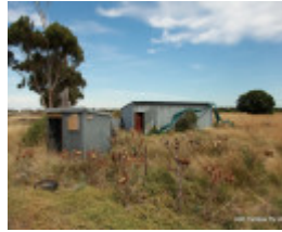
Clean-up re. asbestos 2012
