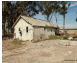
Clean-up re. asbestos 2012
