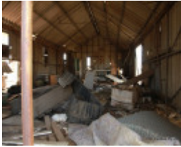
Clean-up re. asbestos 2012
