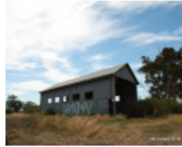
Clean-up re. asbestos 2012
