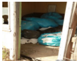
Clean-up re. asbestos 2012
