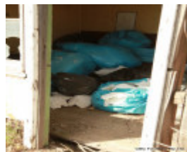
Clean-up re. asbestos 2012
