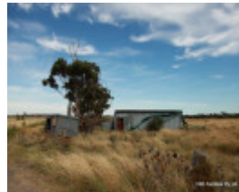
Clean-up re. asbestos 2012
