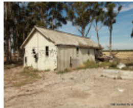
Clean-up re. asbestos 2012
