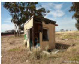
Clean-up re. asbestos 2012
