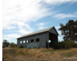
Clean-up re. asbestos 2012
