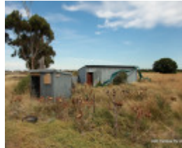
Clean-up re. asbestos 2012
