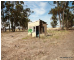
Clean-up re. asbestos 2012
