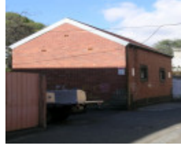
15A McIlwraith Street
