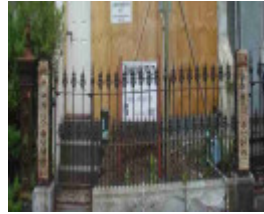
Fence - 746 Drummond Street
