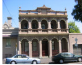
Brassey House Chapman Street North Melbourne March 2006
