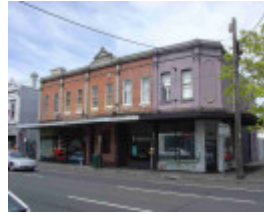
Collingwood Johnston Street 159-167.JPG
