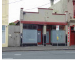
Collingwood Johnston Street 160-162.JPG
