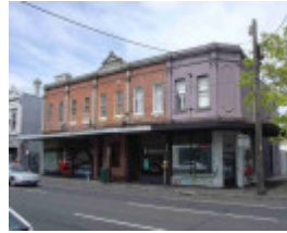
Collingwood Johnston Street 159-167.JPG
