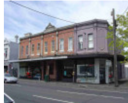
Collingwood Johnston Street 159-167.JPG
