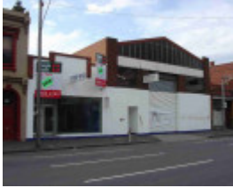
Collingwood Johnston Street 170-176.JPG
