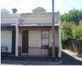
carlton north hughes street carlton north hughes street 8
