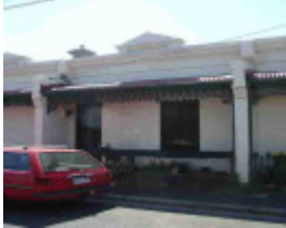
carlton north hughes street carlton north hughes street 12
