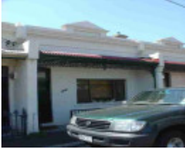
carlton north hughes street carlton north hughes street 16
