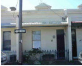
carlton north hughes street carlton north hughes street 18
