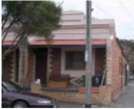
carlton north ogrady street carlton north ogrady street 16
