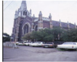
presbyterian church north melb exterior front
