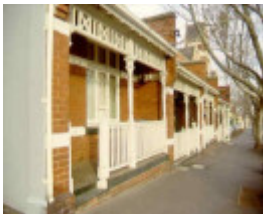
presbyterian union memorial church north melb queensberry street cottages sw aug1999
