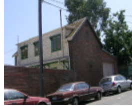
Rear of 23 Clifton Street.JPG
