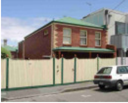
richmond dando street richmond dando street 6
