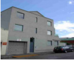
richmond dando street richmond dando street 10
