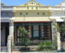
carlton north davis street carlton north davis street 9
