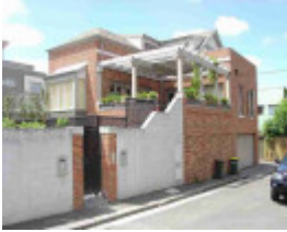
richmond portland street richmond portland street 5
