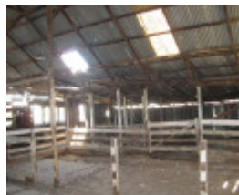
Clonard homestead complex_milking/shearing shed interior
