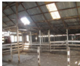
Clonard homestead complex_milking/shearing shed interior
