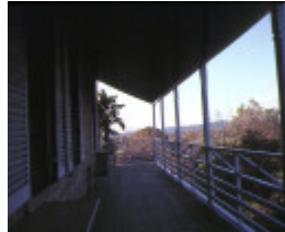
the hermitage murray valley hwy barnawartha view of verandah
