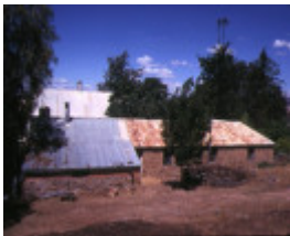
the hermitage murray valley hwy barnawartha outbuildings
