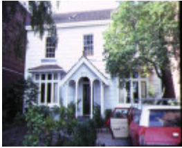
1 456 victoria street nth melb front view
