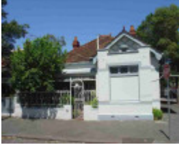
carlton north park street carlton north park street 476
