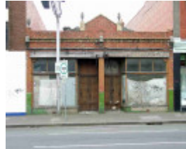
Collingwood Johnston Street 174-176.jpg
