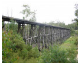
General view of bridge, Jan 2008.
