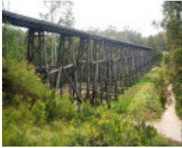
RAIL BRIDGE SOHE 2008
