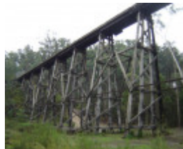
General view of bridge, May 2007.
