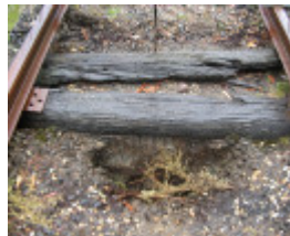
Rails and sleepers detail, Jan 2008.
