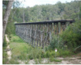
RAIL BRIDGE SOHE 2008
