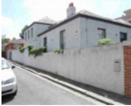
richmond portland street richmond portland street 3
